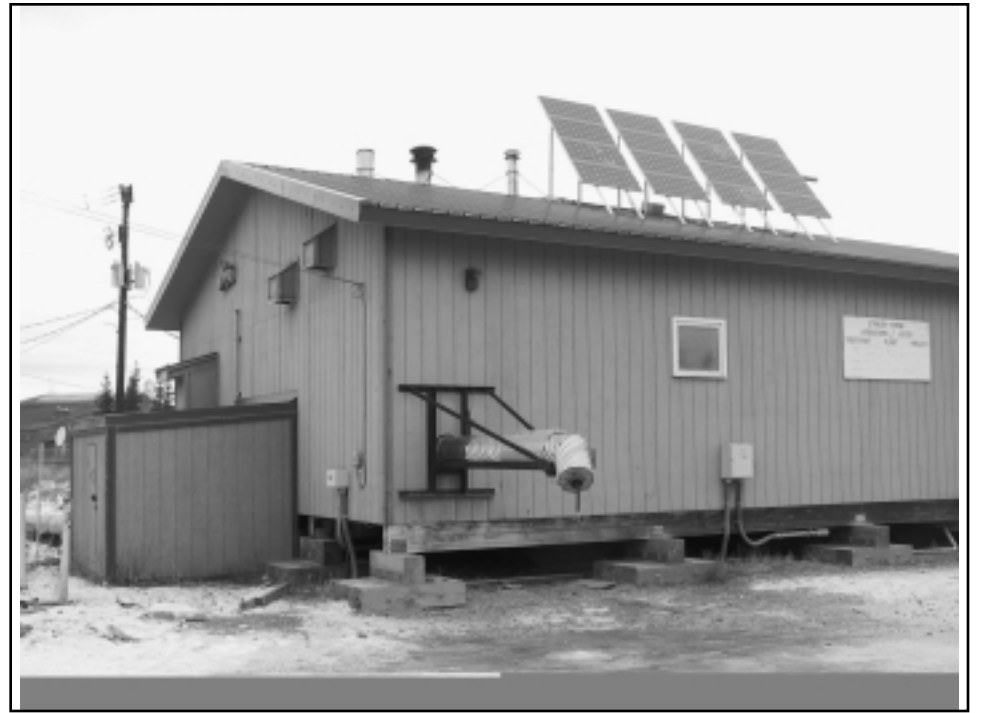
Photo by Scott Henrickson/DEHE staff Venetie's Stanley Frank Washeteria shown with the fixed array, photovoltaic solar panels mounted on the roof.
