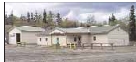
Aleknagik's clinic with emergency response vehicle storage garage.
