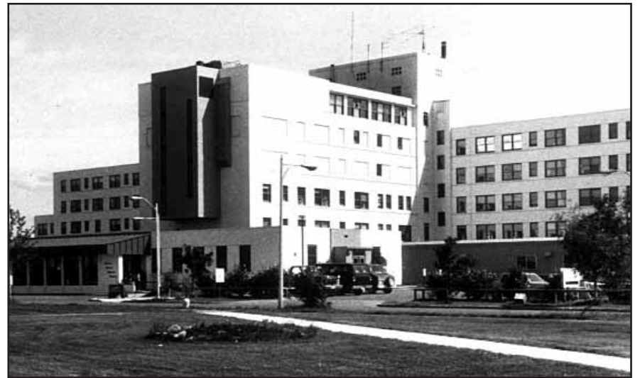
Alaska Native Services was built in 1953 as a tuberculosis sanitarium. As new medications cut TB rates, it became a hospital. The original design, however, made it hard to refit it for new uses.
