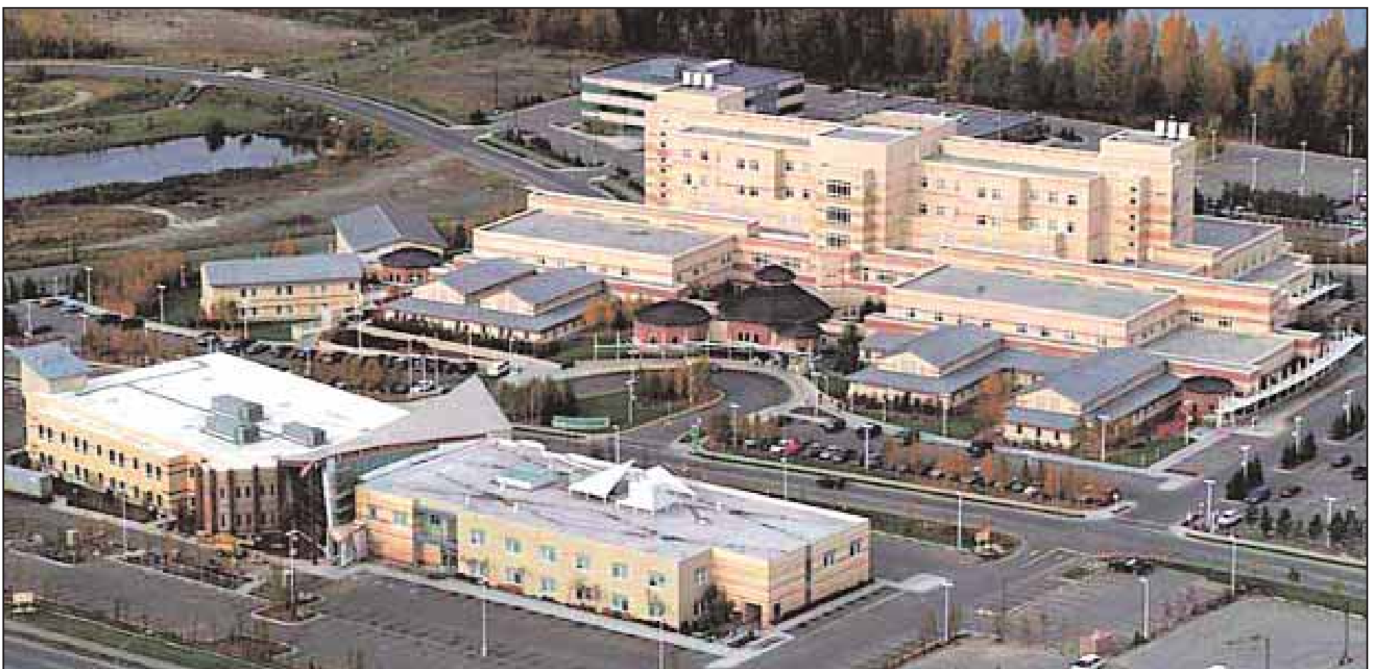
The architectural firm NBBJ designed the new Alaska Native Medical Center with the help of an Elders' Advisory Committee. Southcentral Foundation selected NBBJ for the expansion of the ANMC Anchorage Primary Care Center (PCC) so that its design would fit with long-term plans for the Alaska Native Health Campus. PCC is shown at the bottom left in this aerial photo.
