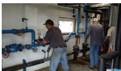
David Walker and Bruce Werba working on changing out the pipes of the Holy Cross Water Treatment Plant
