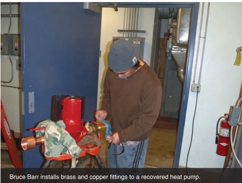
Water plant operator Bruce Barr prepares a copper pipe for sweating to a recovered heat pump in Deering.
