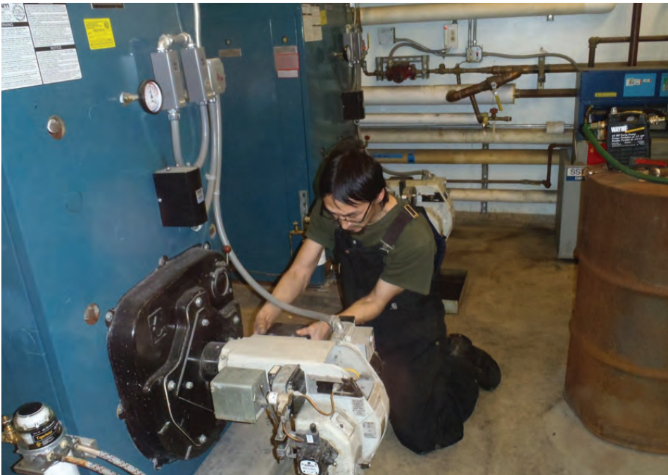
Deering water plant operator Fletcher Gregg installs energy efficiency upgrades on the oil-fired boiler in the community's water plant and washeteria.
