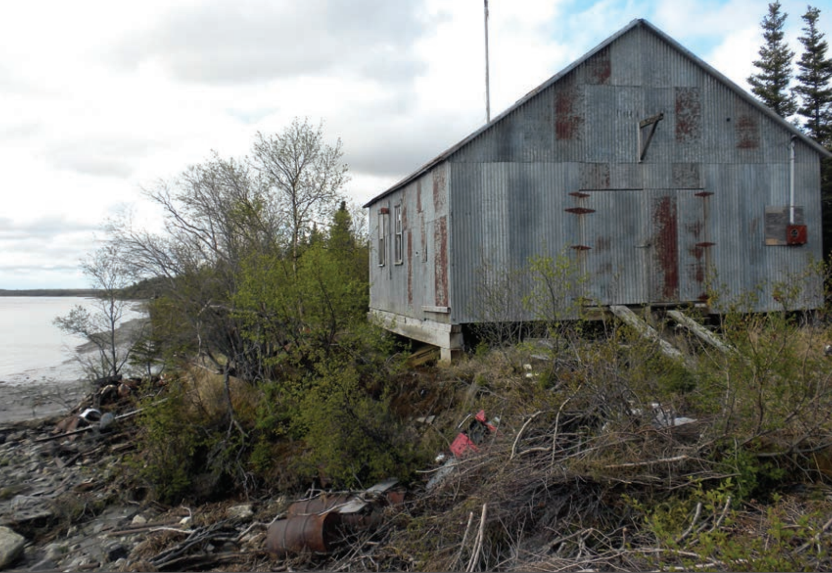
Erosion threatens old warehouse. Mike Brubaker, 2013.
