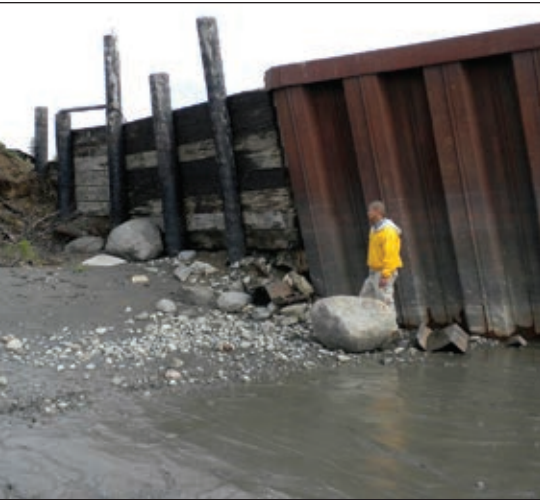
Erosion of the community bulkhead. Mike Brubaker, 2013.
