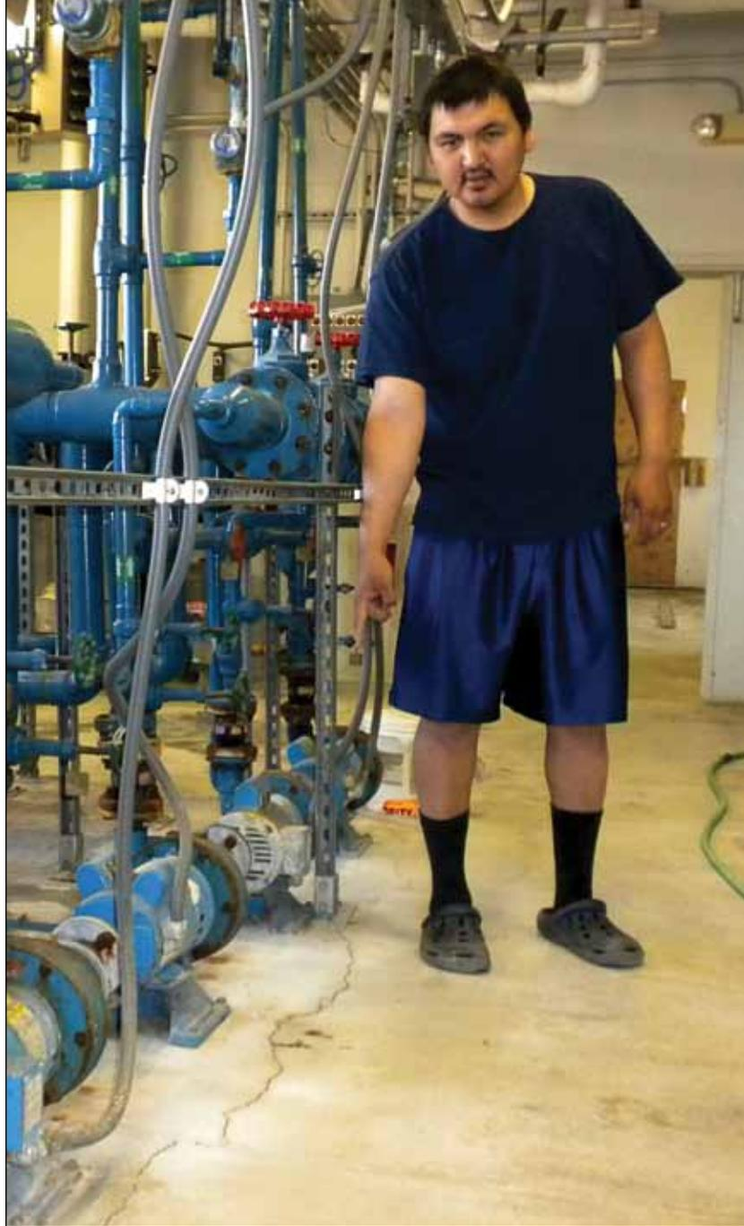
*Jeffery Luther shows foundation crack in water plant.
