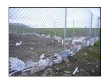
Site was prepared for fencing. A bulldozer was used to push trash into a trench, compact, then cover with soil to help minimize the smell & the workers contact with potential hazards. Scattered trash was cleaned up along fence post diameter.
