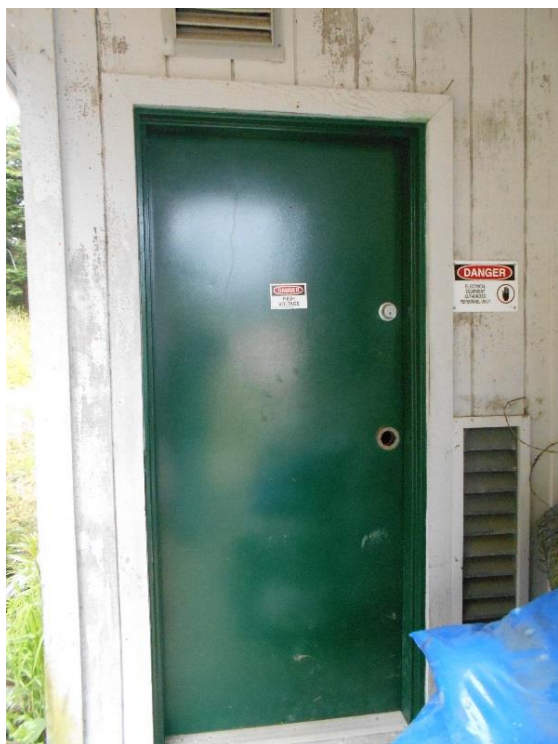
Figure 3.6: Generator Room door with no doorknob.
