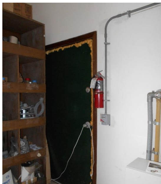
Figure 3.7: Chemical Room door with foam insulation sealing the spaces around the door frame.
