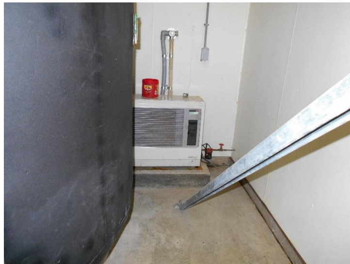
Figure 3.9: Toyotomi Laser 73 in the process room of the water treatment plant. This unit is not used.
