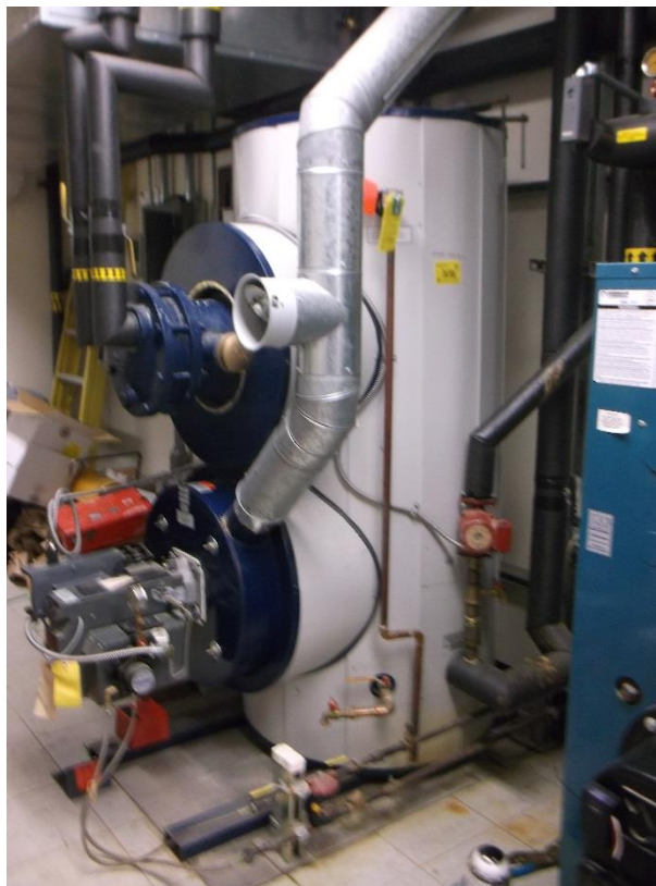
Figure 3.5: Hot water heater in the Golovin Washeteria
