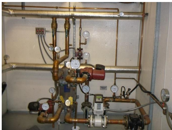
Figure 6: Heat Recovery System in the Golovin Power Plant
