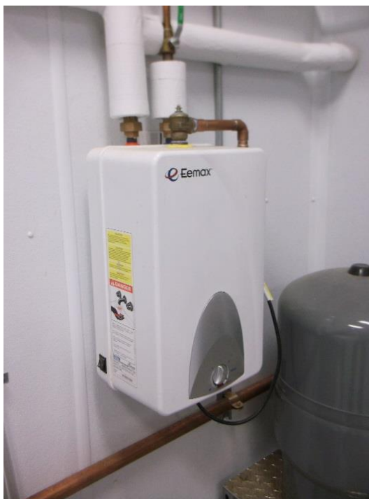
Figure 3.3: Electric Hot Water Heater
