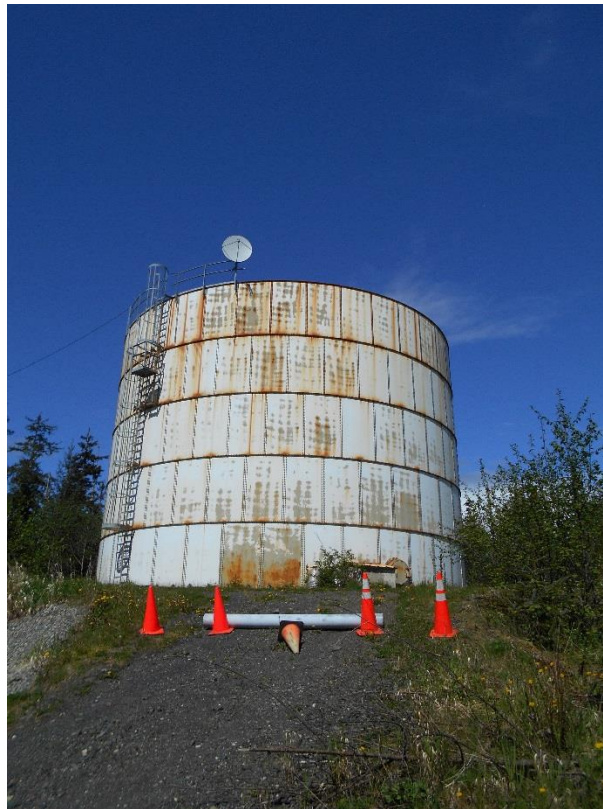
Figure 3.1: The 375,000 gallon water storage tank at the water treatment plant site.
