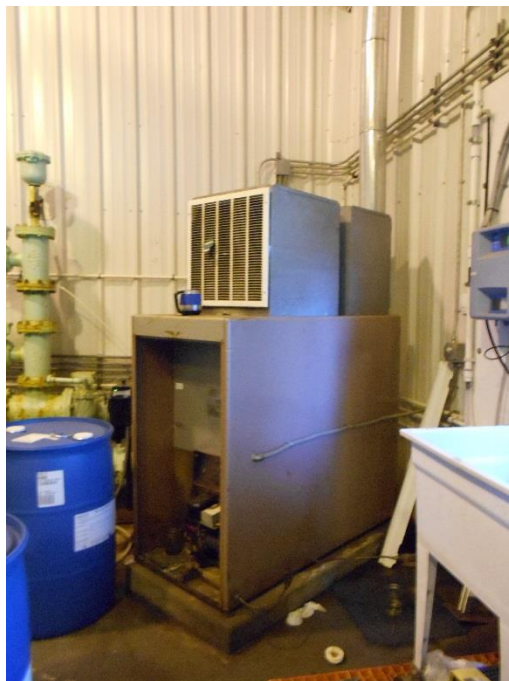
Figure 3.9: Oil-fired Space Heater in the Water Treatment Plant Process Room.
