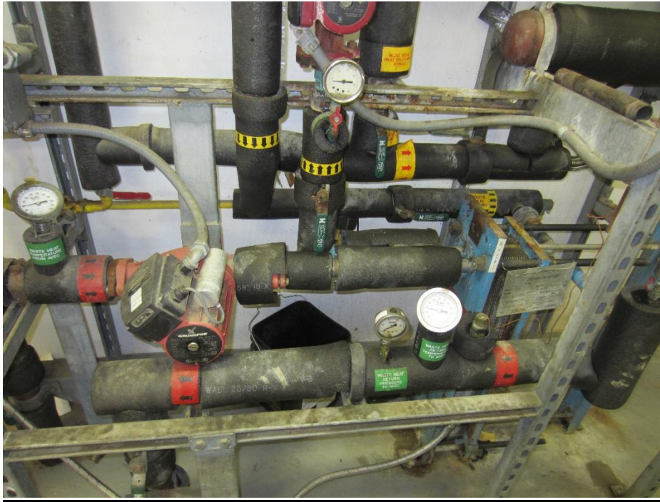
Figure 3: Heat recovery; heat exchanger where heat from the power plant loop is transferred to the WTP loop.
