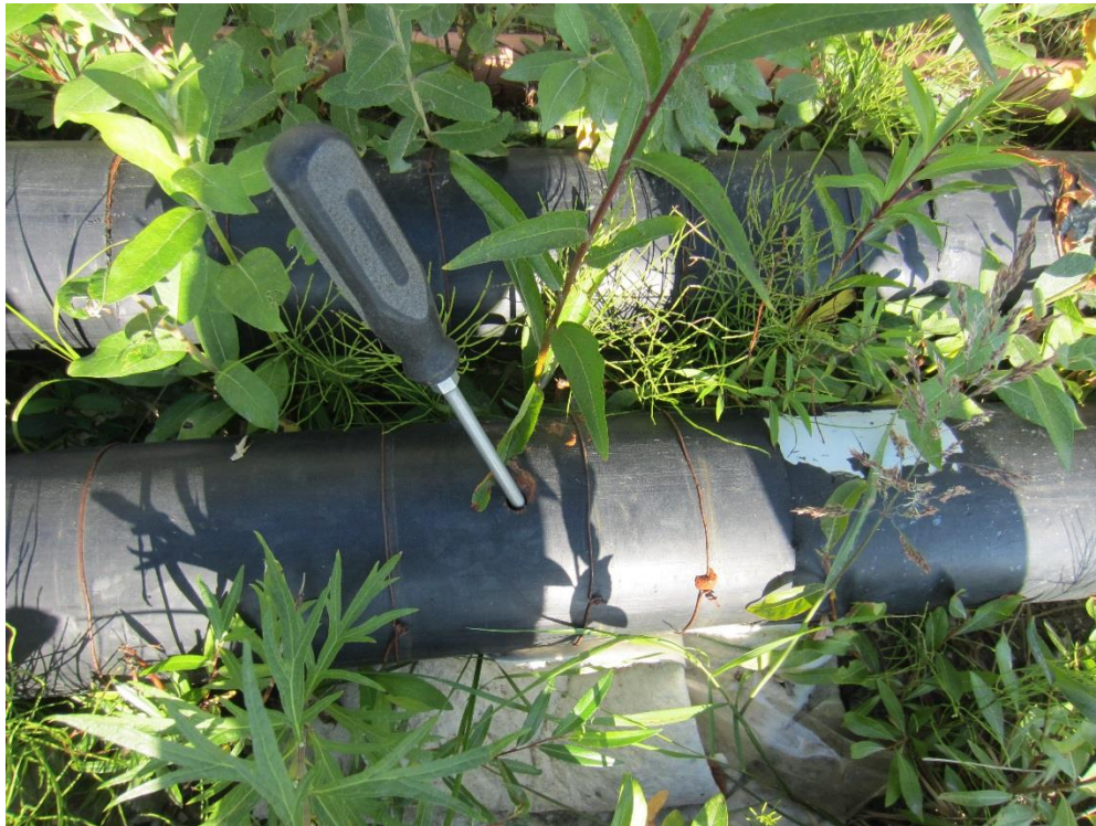
Figure 4: Holes and missing insulation on heat recovery pipes.
