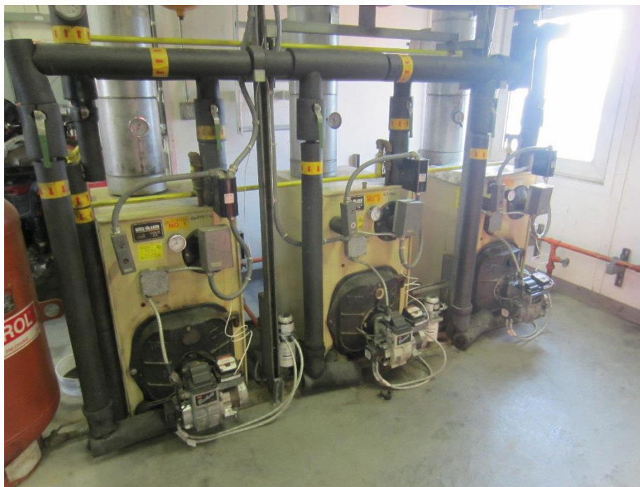
Figure 2: Existing fuel oil boilers.
