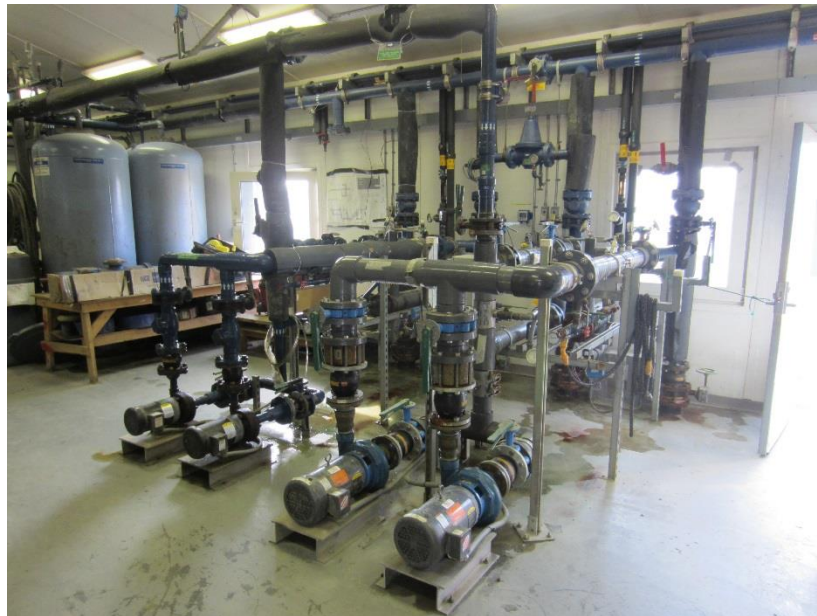
Figure 1: Pressure tanks and circulation loop components in Kiana WTP
