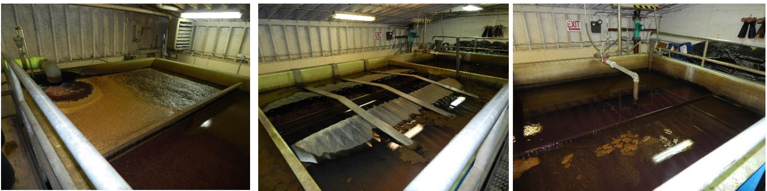
Figure 2: Three photos showing one of two open filter process tanks.
