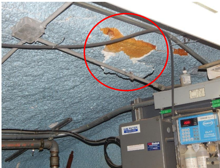
Figure 6: Pieces of insulation are falling off from the ceiling by the raw water intake.
