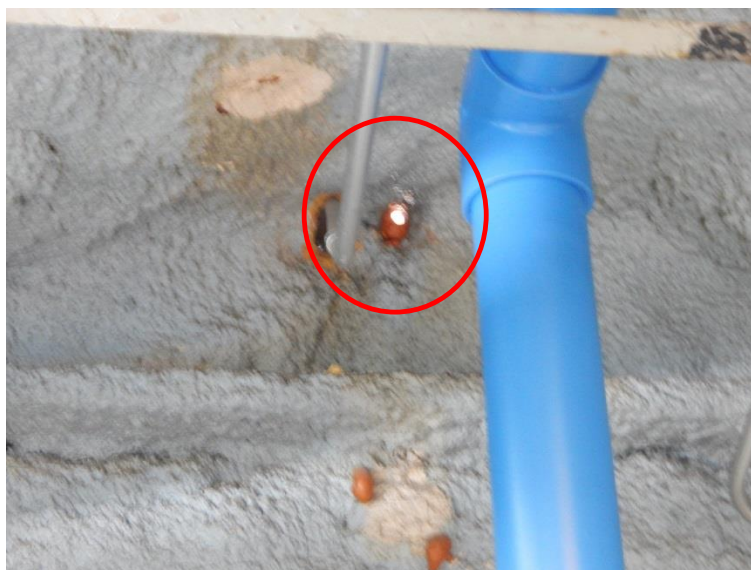
Figure 4: Visible holes in the wall insulation where air can leak directly to the outside.
