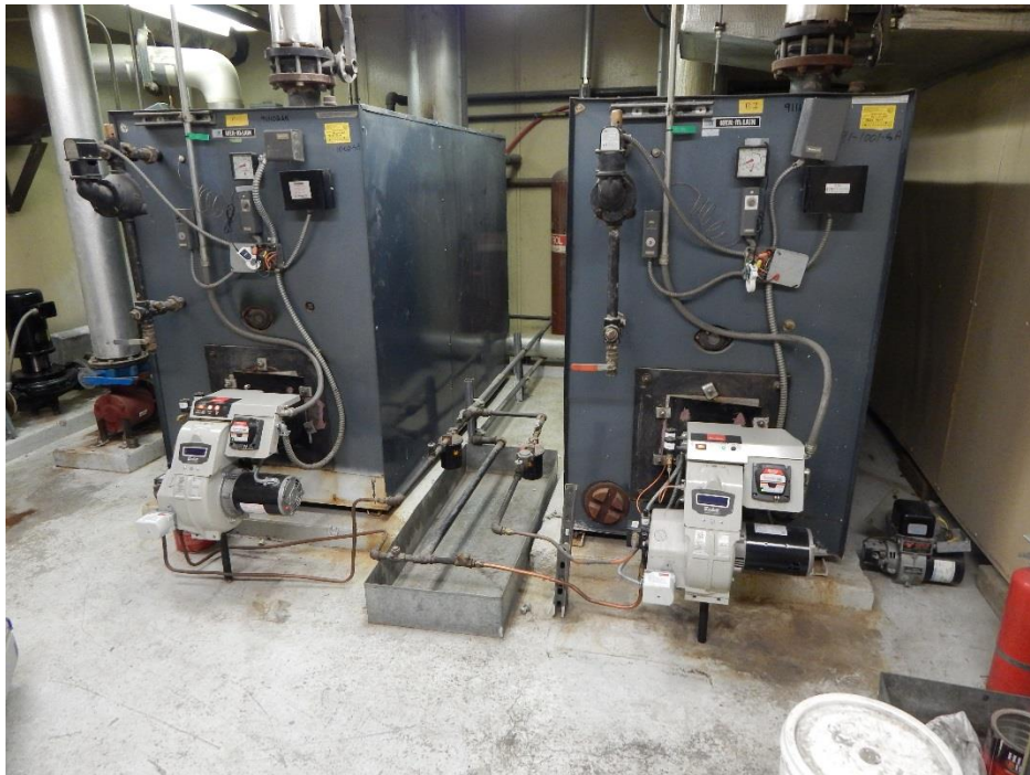
Figure 9: Weil McLain boilers in the boiler room. These boilers are used for the space heating in the building.
