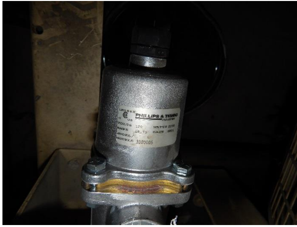
Figure 10: Generator Block Heater
