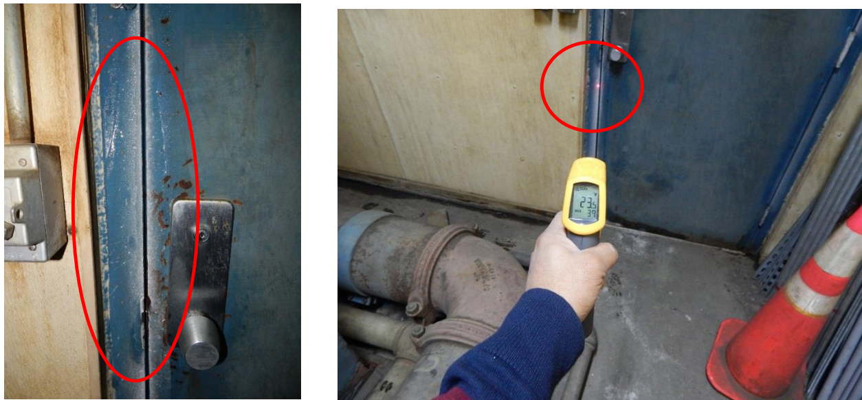
Figure 11: Two photos showing the filtration room door seam with ice buildup due to the humidity from the filters. As a result of poor insulation and excessive air infiltration, the temperature at the door seam was 23 deg. F.
