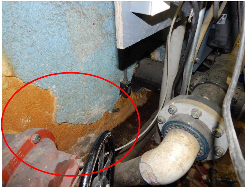
Figure 3: Insulation damage on the wall near the water storage tank wall penetrations.
