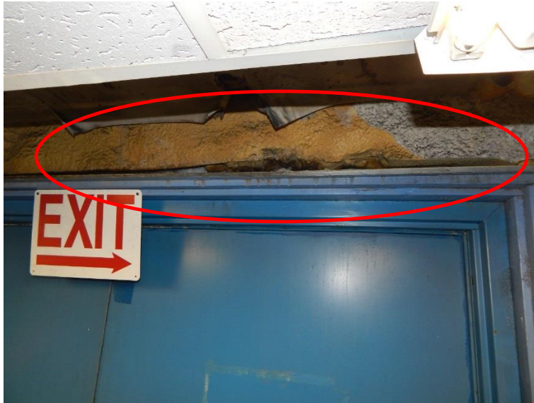
Figure 5: Insulation damage along the door seam by the process room doors.
