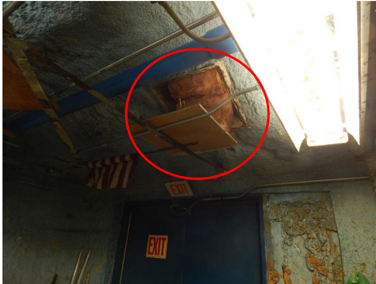
Figure 7: A panel of insulation is falling through the ceiling of the building.
