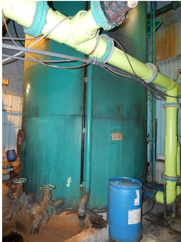
Figure 1: Surge Tank used for mixing Aluminum Sulfate Hydrate into the water.
