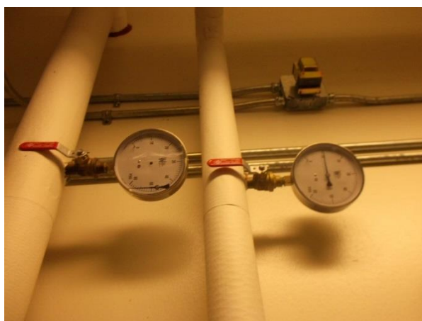
Figure 7: Broken Gauges within the Mechanical Room
