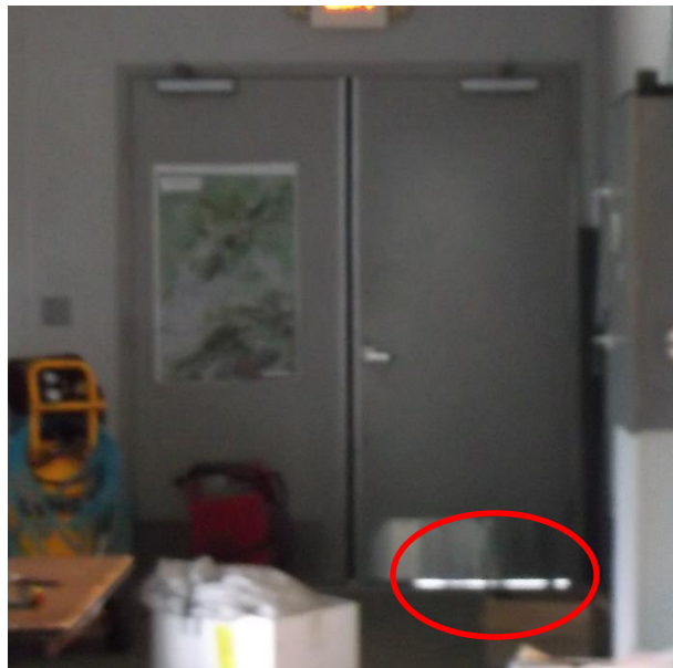
Figure 2: Door in Water Treatment Plant, needs to be weatherized
