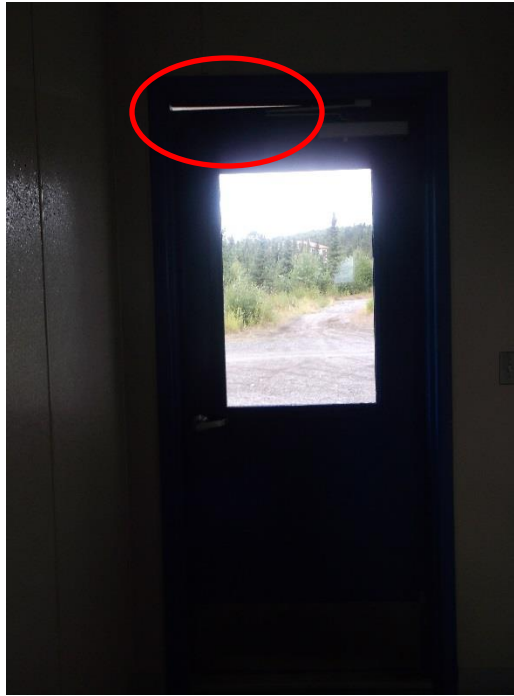
Figure 1: Door in Artic Entry, needs to be weatherized
