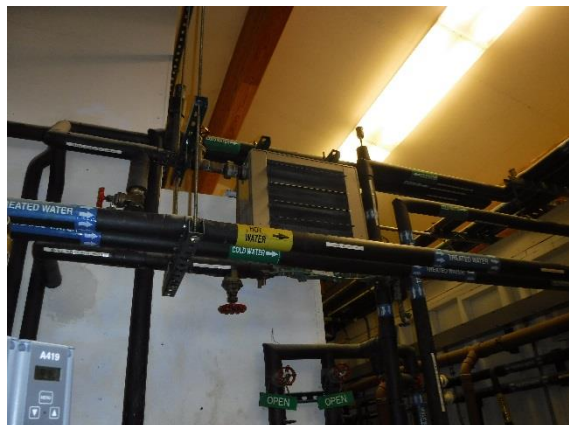
Figure 9: Process Room Unit Heater
