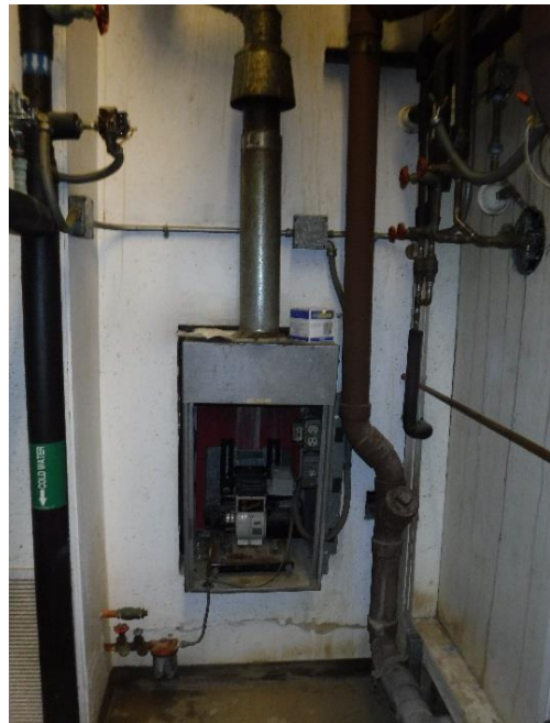
Figure 4: Sauna Heater Blower Unit
