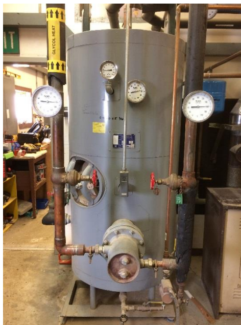
Figure 8: Fuel Oil Hot Water Heater
