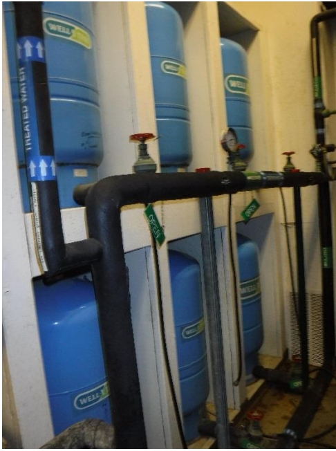
Figure 1: Pressure Tanks used for Water Storage
