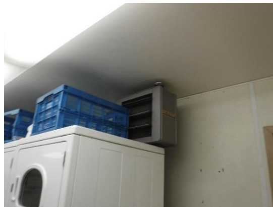
Figure 10: Washeteria Unit Heater
