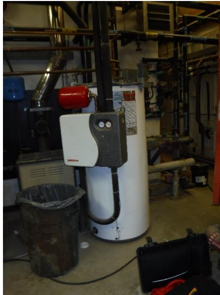
Figure 7: Solar Thermal Water Heater
