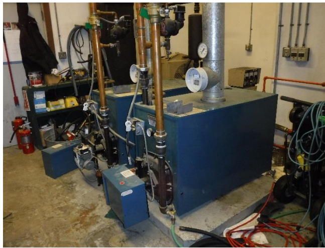
Figure 6: Fuel Oil Boilers
