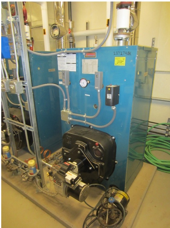
Figure 3: The boilers and heat recovery heat exchanger in the Buckland Water Treatment Plant.
