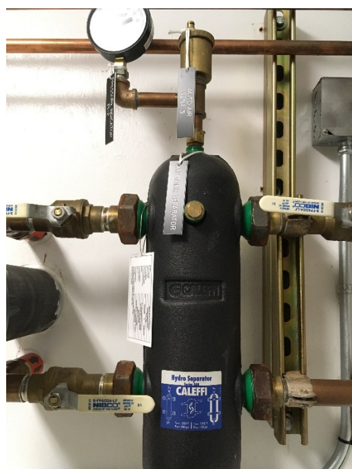
Figure 5: The “decouple” that hydraulically connects the heating lines in the WTP and pump house.
