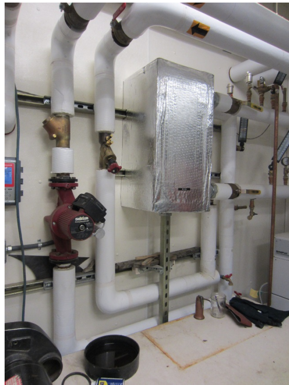
Figure 3: The boilers and heat recovery heat exchanger in the Buckland Water Treatment Plant.
