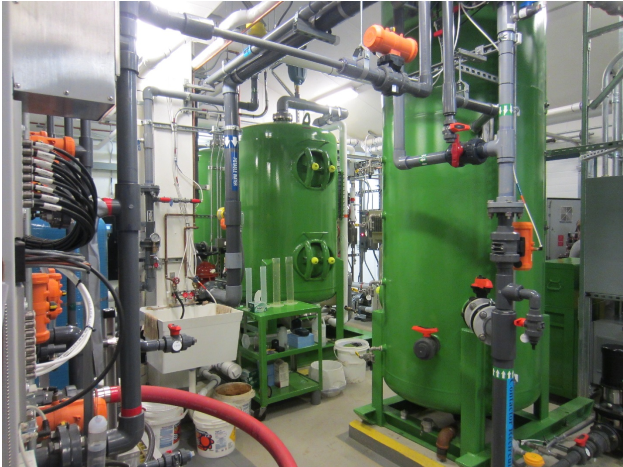
Figure 2: Filters and the MIEIX contactor tank in the main room of the Buckland Water Treatment Plant.
