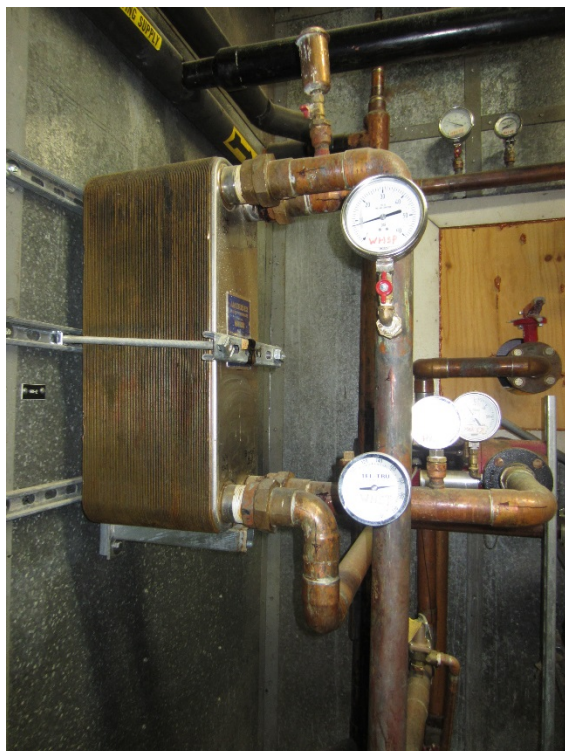
Figure 4: Heat recovery system heat exchanger in washeteria boiler room.
