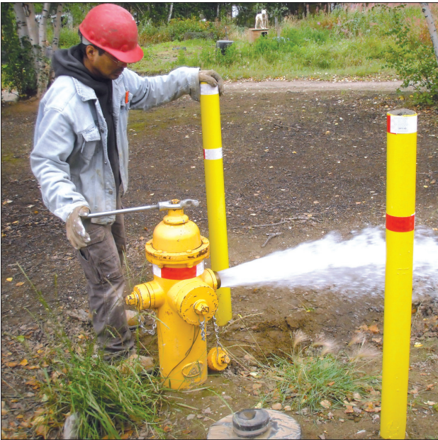
PHOTO BY ANTHC Workers test a flush hydrant in Huslia, where ANTHC teams are completing a multi-year water main replacement project.
