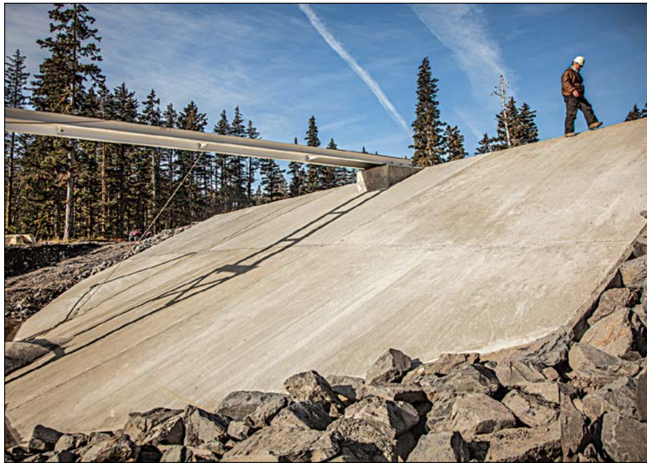
PHOTOS BY CLARK JAMES MISHLER ANTHC staff examines the new community dam of Ouzinkie, which recently began operation.
