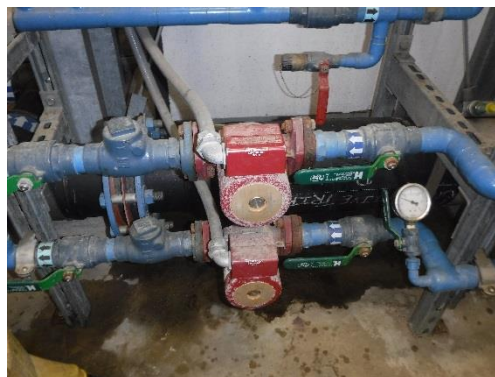
Figure 13: Heat-add circulation pumps with visible corrosion.
