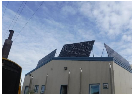
Figure 9: Solar photovoltaic system on the water treatment plant
