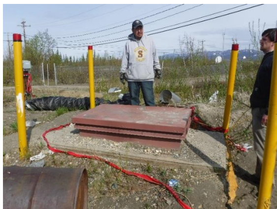
Figure 2: Upper vault of river intake system.
