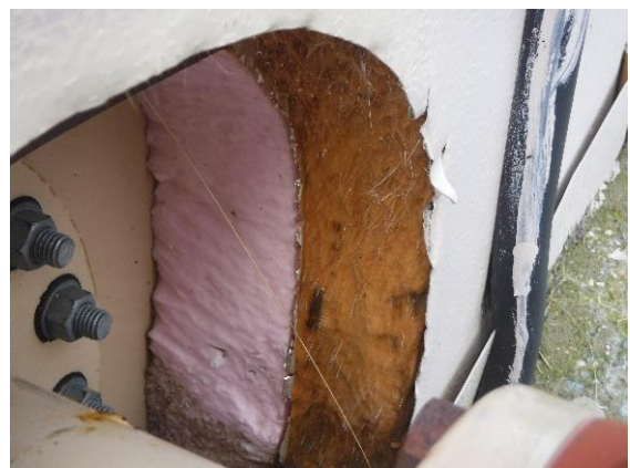
Figure 6: Water storage tank insulation
