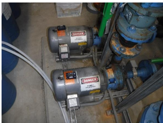
Figure 14: Pressure pumps
