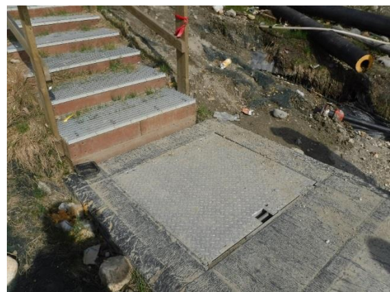
Figure 3: Lower vault of river intake system.
