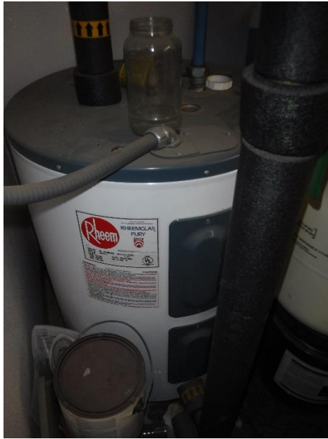
Figure 11: Electric hot water heater
