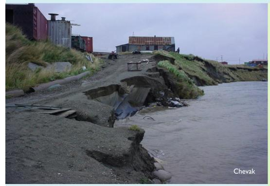
Chevak homes and roads are threatened by river erosion and permafrost melt. Sink holes are appearing throughout in the community.
