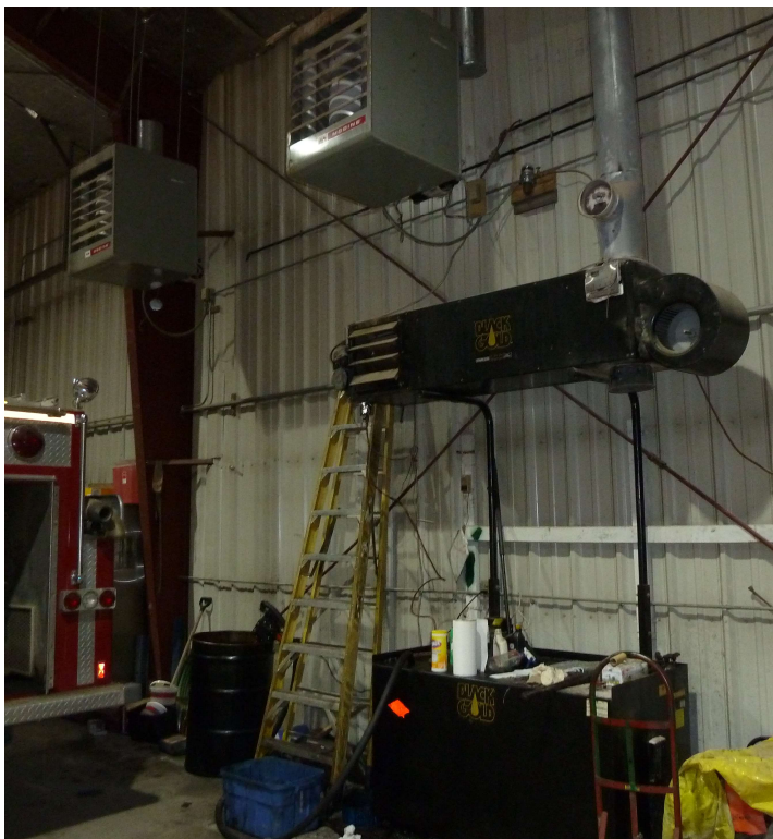
Waste oil burner and both oil fired unit heaters, 1 of which appears to be functional (and was running during the site survey)
