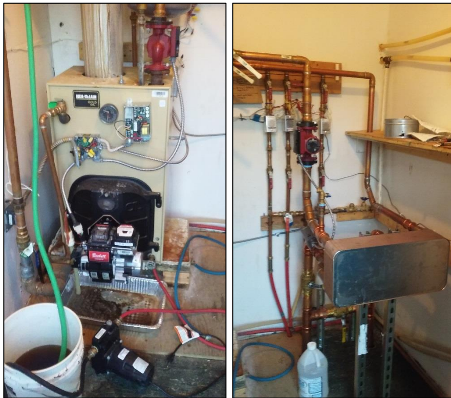
Figure B2. Community Hall boiler (left) and district heating heat exchanger (right).
