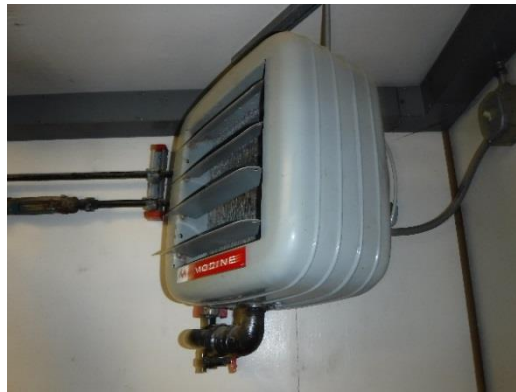
Figure 9: Water Treatment Plant Unit Heater
