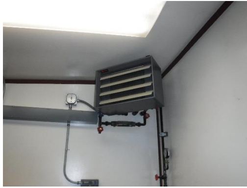
Figure 8: Generator Room Unit Heater
