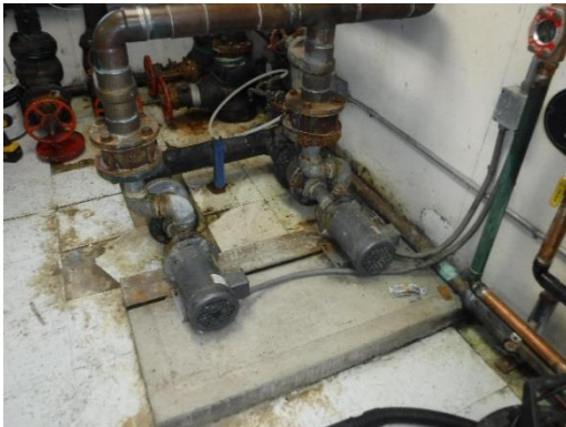
Figure 12: Water Circulation Pumps
