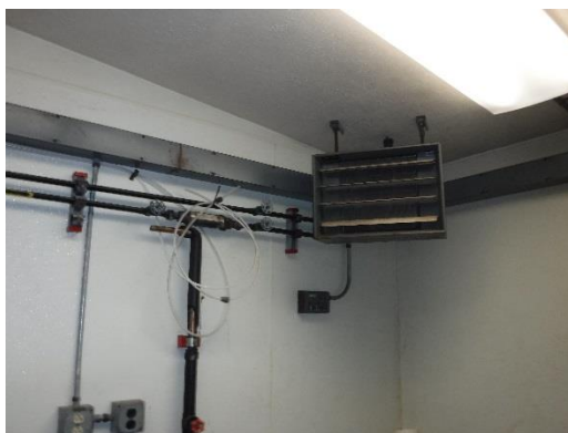
Figure 7: Storage Room Unit Heater
