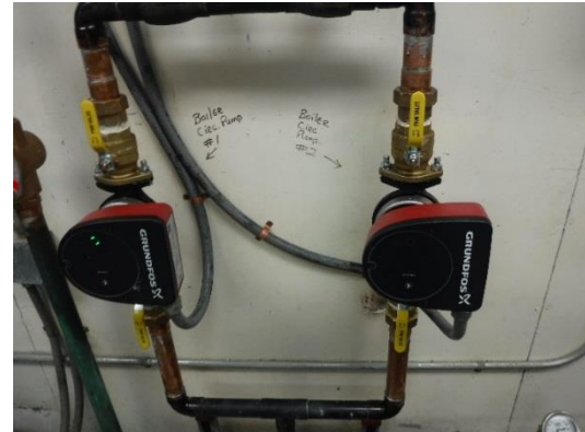
Figure 11: New Glycol Circulation Pumps
