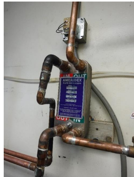
Figure 13: New Water Circulation Heat-Add Heat Exchanger
