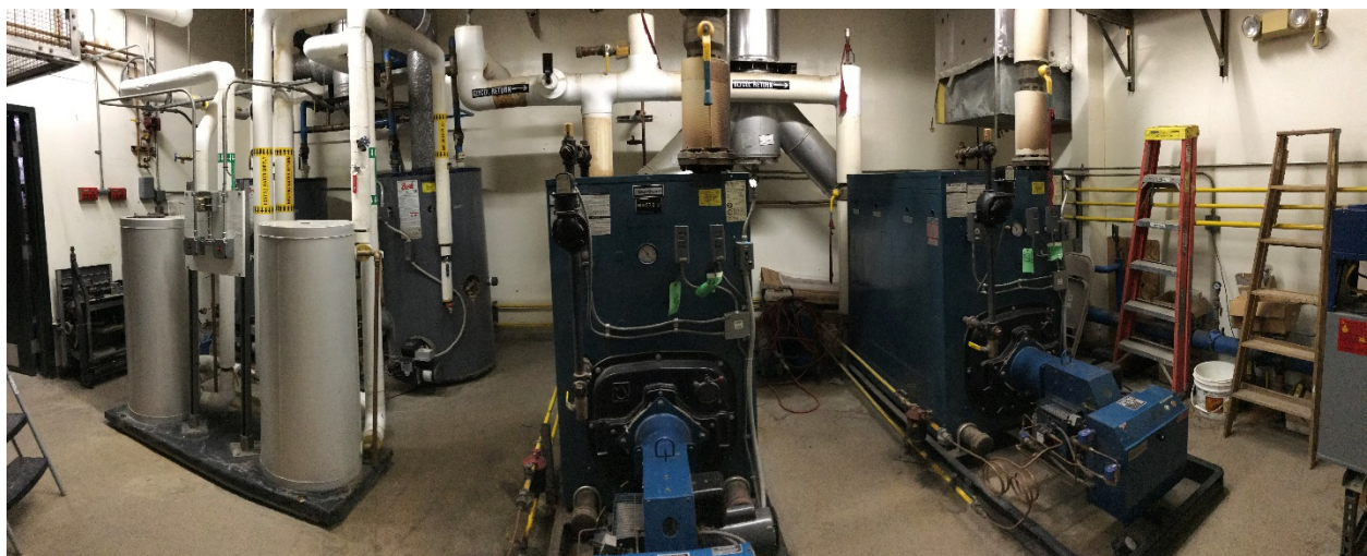
Figure 5: Left: The WTP/Laundromat Boiler Room. The white hot water generators on the left are served by the wood boilers. The older gray hot water generators behind them now serve as hot water storage tanks.
