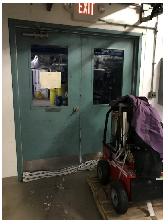
Figure 3: Rags are used to mitigate air leakage under the process room doors.
