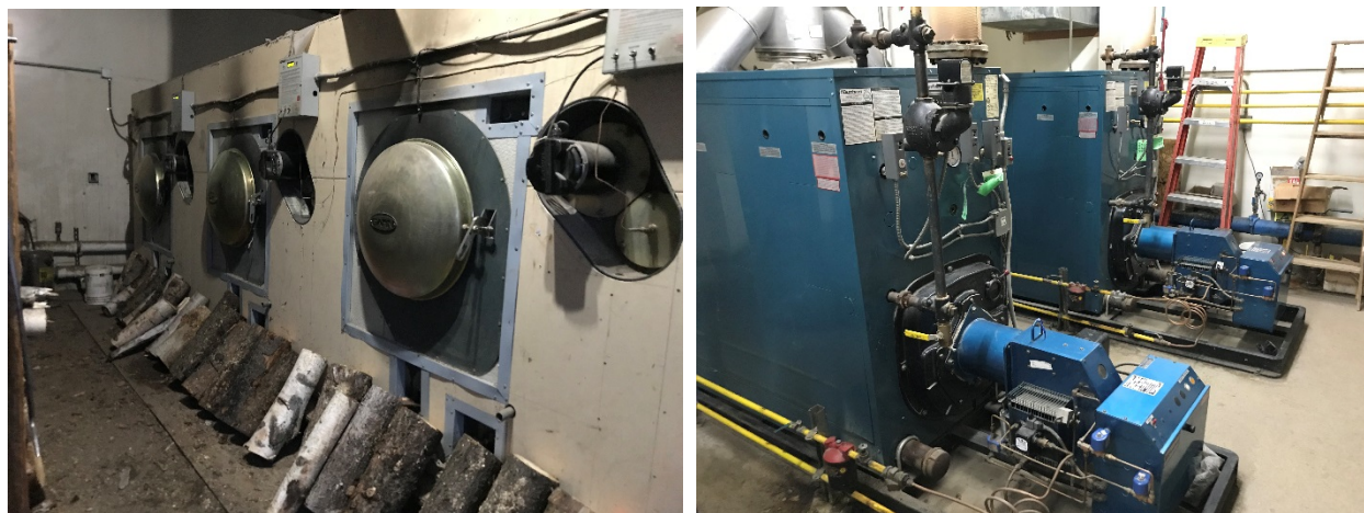
Figure 4: Left: Garn wood boilers located in the city garage behind the Laundromat. Right: Burnham oil-fired boilers located in the WTP.
