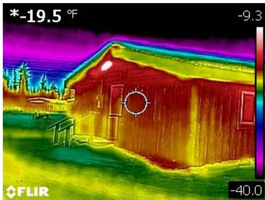
FLIR thermal imaging of the building rear exit. The color gradient on the right depicts the temperature range of the photo (-40° F to -9.3° F).
