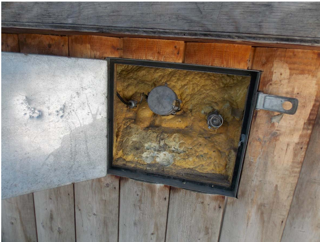
Sewage tank outlet and exterior insulation.
