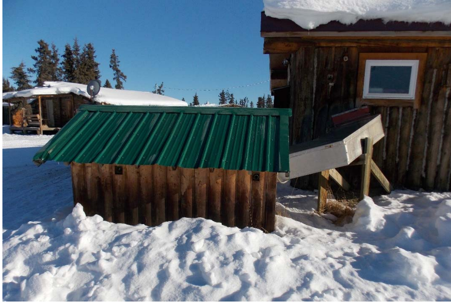
Flush/haul system “dog house” sewage tank on the exterior of the Head Start Building. Electric heat trace runs down through the discharge pipe and along the bottom of the holding tank.
