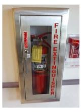
Generally, a person should not need to travel more than 30 feet to access an extinguisher. Check the front label to ensure the operating instructions are in place and visible. If tamper seals are used, check the tamper seal.
