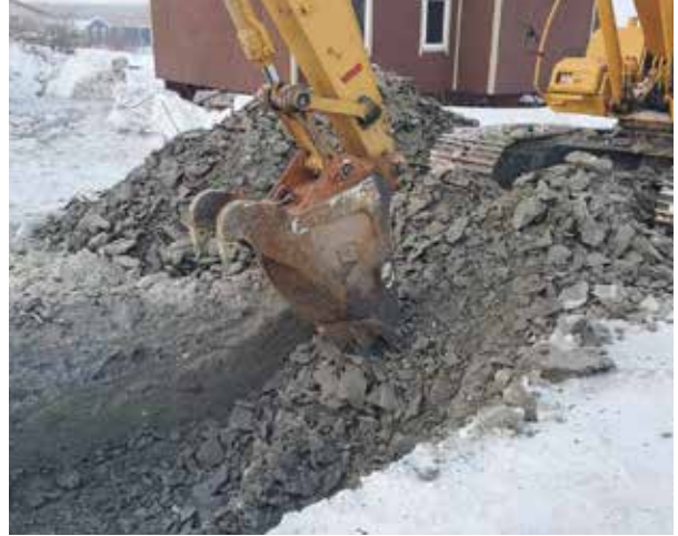
Kiana Pressure Pump Upgrades Installation
