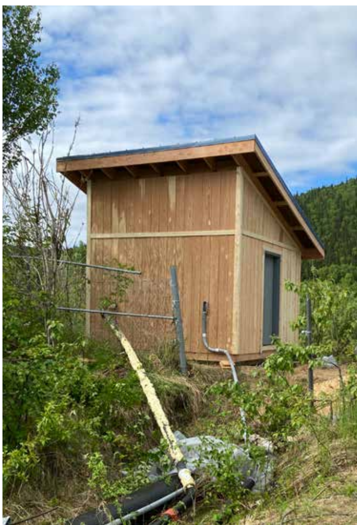
Upper Kalskag Pump House
