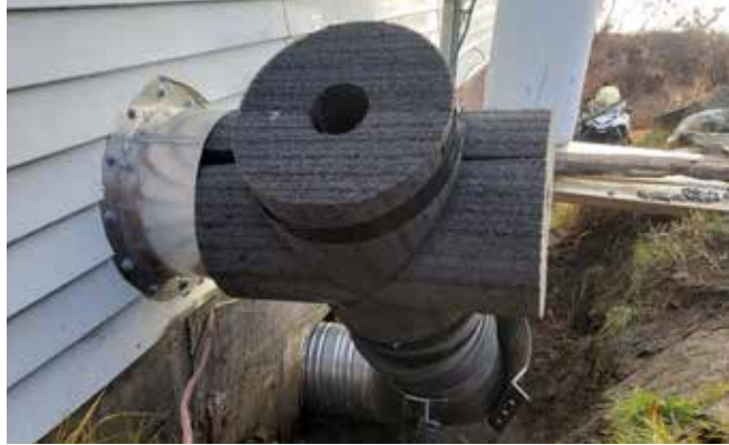
Golovin Water and Sewer Installation
