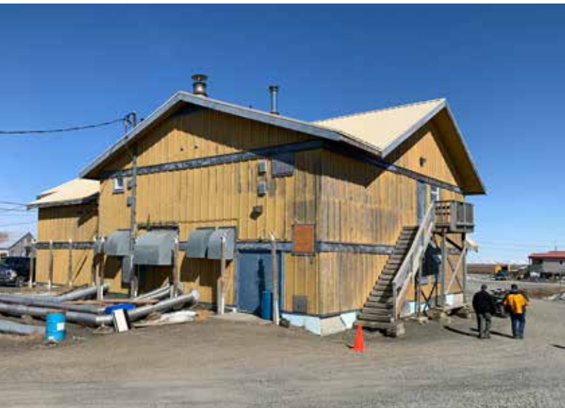
Quinhagak Structural Engineering Water Treatment Plant Assessment
