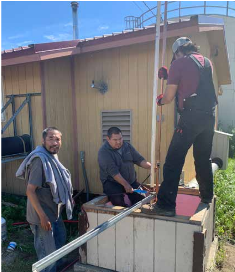
Kobuk Well Inspection
