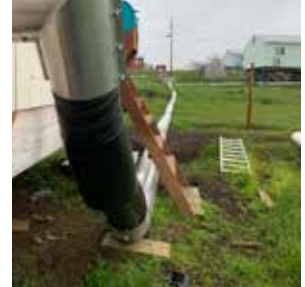
Chevak Service Line Installation
