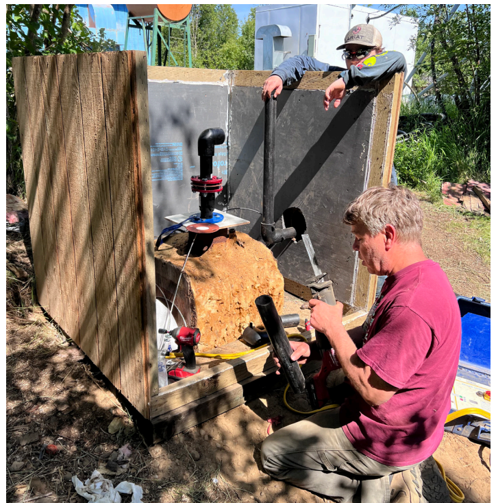
New Stuyahok Temporary Water Line
