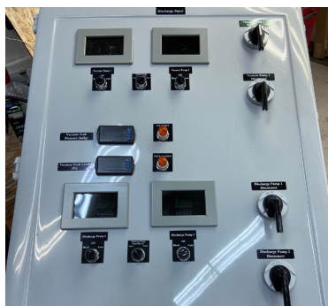
Deering Vacuum Discharge Panel
