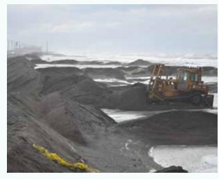
**Figure 44:** A five mile gravel berm provides insufficient shoreline protection from coastal erosion in Utqiagvik and must be repaired after every storm, as shown above, which costs \$8.3 million annually. The U.S. Army Corps of Engineers project will construct a fortified rock revetment to protect the shoreline. **Credit:** North Slope Borough.
