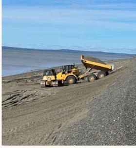
**Figure 22:** Shaktoolik's storm surge berm in August 2022, shortly before the Merbok storm. **Credit:** ANTHC.
