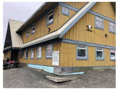
**Figure 24:** The exterior walls of the Quinhagak multi-purpose building have settled relative to the interior and the floor tilts 9 inches to the southwest over a horizontal length of 22 feet. There is widespread damage, including a three-inch crack between the wall of the health clinic and the floor. Short-term stabilization is recommended. The long-term solution is to replace the building. **Credit:** Chinik Eskimo Community; 2005.
