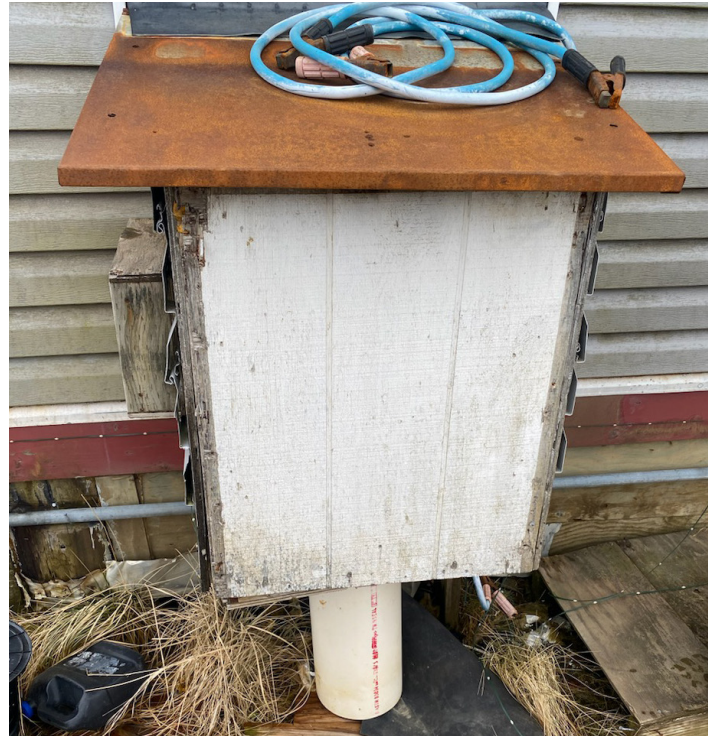
New Stuyahok Arctic Box Repairs
